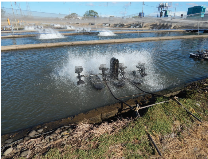
FIGURE 5. Aeration of intensive flow-through tilapia ponds operated by ACI.
