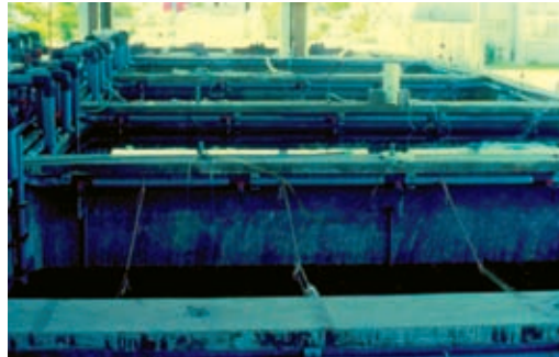
Fig. 12. Concrete larval rearing tanks, each 50 m 2 , in Japan. (Photo by John Tucker)
