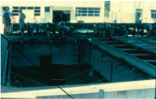
Fig. 13. A 50-m 2 concrete larval rearing tank in Japan (from the group in Fig. 12). (Photo by John Tucker)
