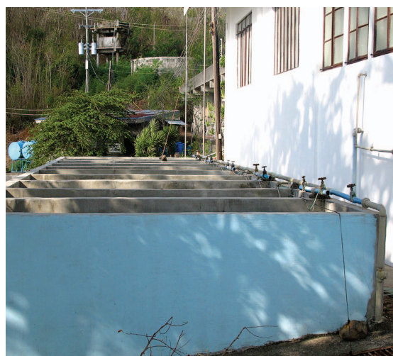
Concrete tanks for tilapia culture at SEAFDEC/AQD, Binangonan Freshwater station, Rizal, Philippines. Photo by J.A. Ragaza.
